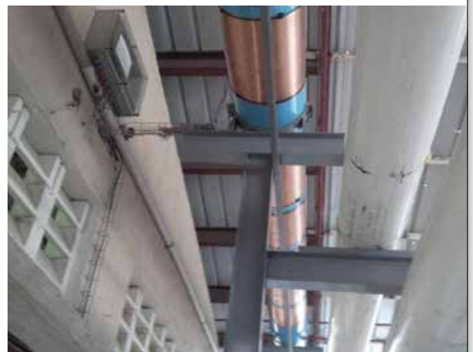
Vulcan S500 cable windings
