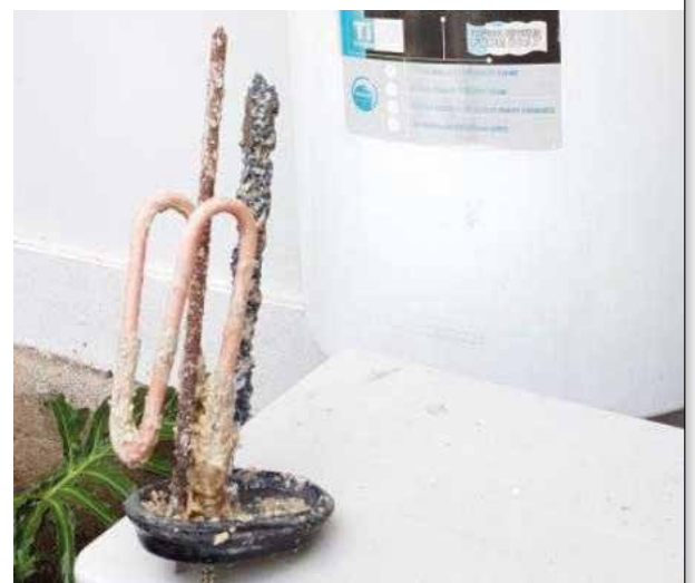
The little remaining scale is soft and easily flushed out since installation of the Vulcan Anti-Scale System.
