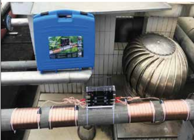
Vulcan S25 was installed on the main water pipe of the guest room Building B.
